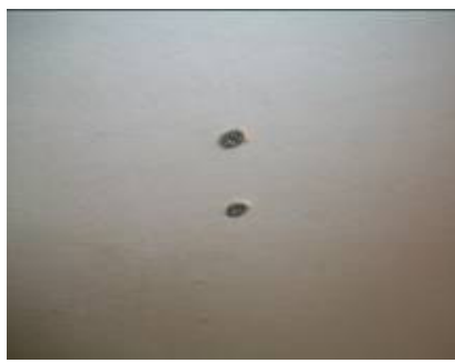
Fitment holes to wall right of entry to bedroom 2
