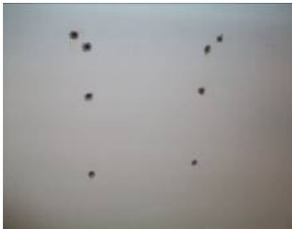
Fitment holes to wall right of fireplace
