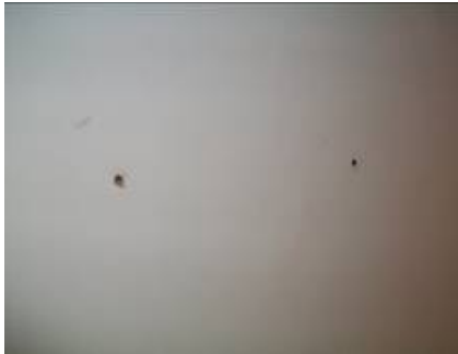
Fitment holes with rawl plugs to wall between wall lights
