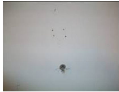
Fitment holes to wall
