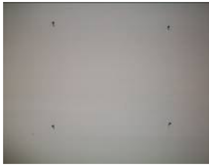
4x nails to wall above toilet
