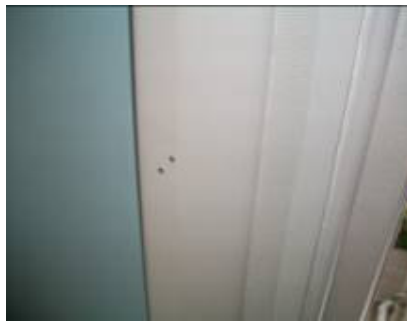
Fitment holes to window frame
