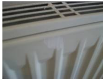
Paint mark to radiator
